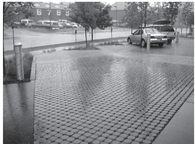
Figure 1-4 Porous paving allows rainwater to percolate rather than run off.
