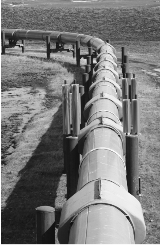
The Trans-Alaskan pipeline.
