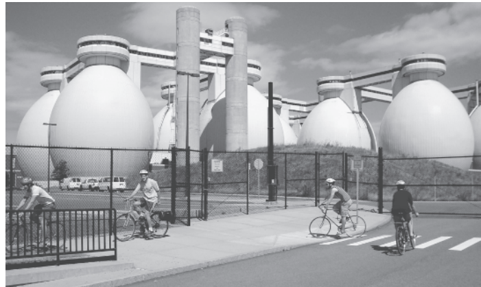
Figure 1.11 Digesters at the wastewater treatment plant Deer Island, MA (Source: Frank Hebbert/Wiki Commons).
