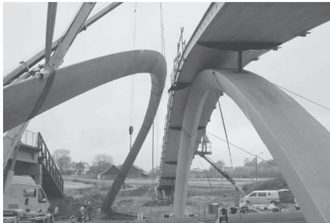
Bridge under construction, 2001, Vebjorn Sand, Norway.
