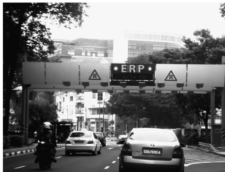
Figure 1.10 Electronic Road Pricing (ERP) gantry in Singapore
