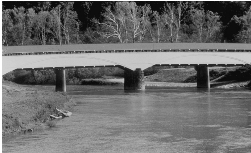
Fig. 1.4 Philippi covered bridge. (Photo by Larry Belcher, courtesy of West Virginia Department of Transportation.)
