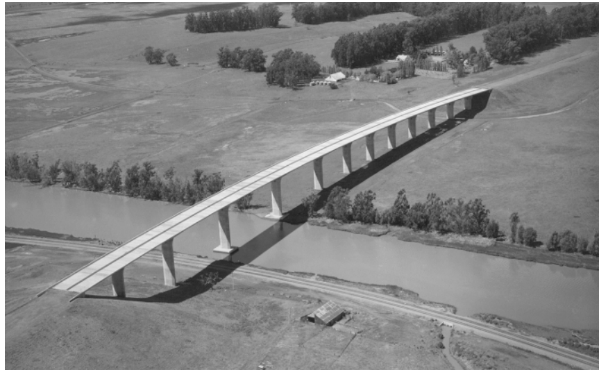
Fig. 1.15 Napa River Bridge. (Photo courtesy of California Department of Transportation.)
