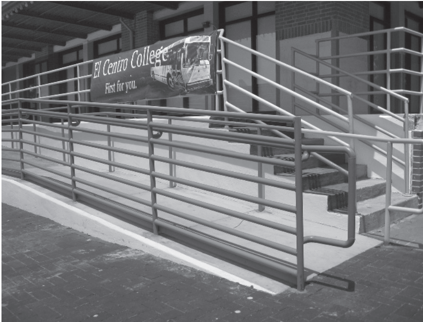
Figure 1.23: A ramp is required when the changes in level exceed ½ inch.
