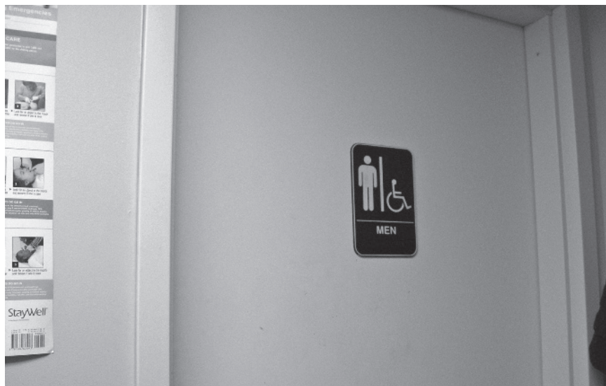
Figure 1.32: This photo shows a sign that is mounted to the pull side of the door where a person could open the door as the visually impaired person is trying to read the sign.
