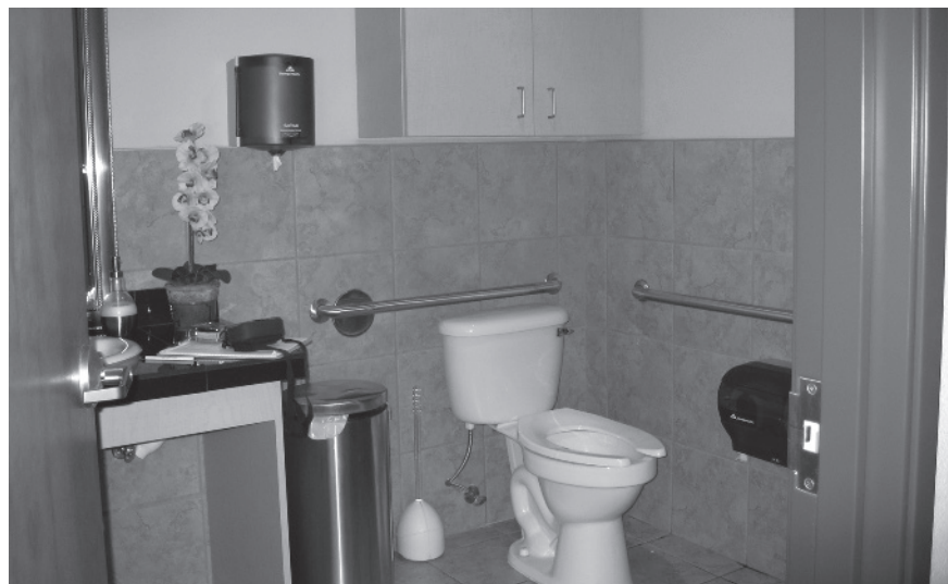
Figure 1.10c: The cabinet located above the toilet does not meet the reach ranges as directed by the ADA Standards.
