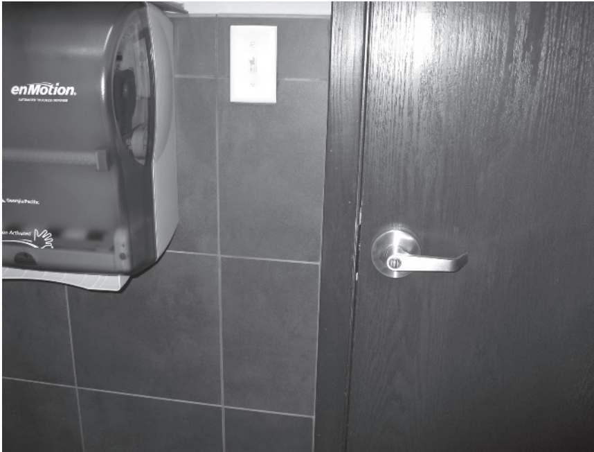
Figure 1.13: This door handle is obstructed by the paper towel dispenser, since it is closer than 18 inches, which prevents a person in a wheelchair from reaching it to open it.
