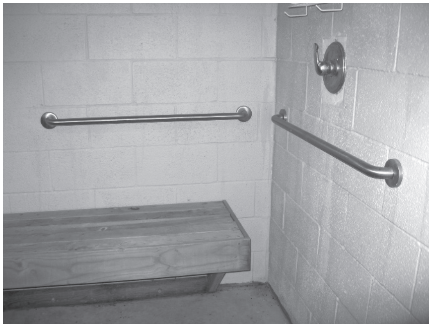
Figure 1.30: This roll-in shower has a seat that is not foldable and is, therefore, an obstruction in the floor space.
