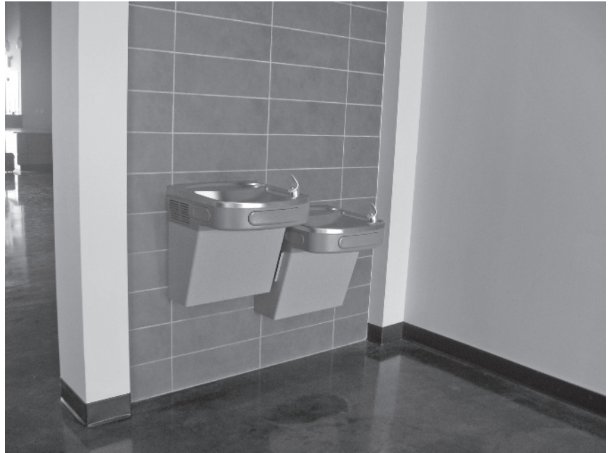
Figure 1.7: This drinking fountain is not located along the main path of travel, but it is a protruding object because it is along a path of travel that a blind person would use.
