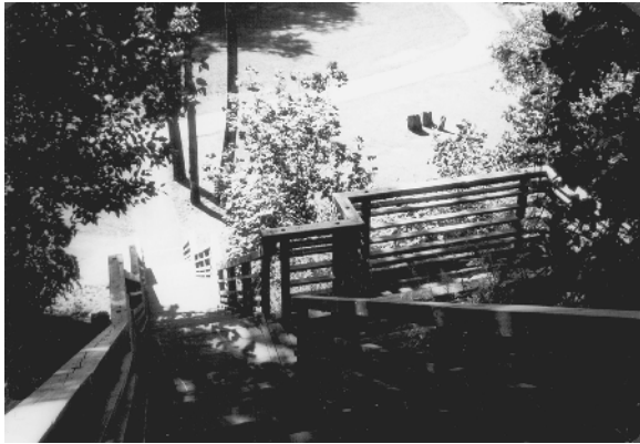
Figure 1.11. Overlook platform at access stair does not interrupt the line of the stair structure.
