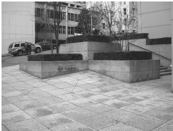
Figure 1.20. The clean, square edges of the planter walls exaggerate an already-steep slope running adjacent to them.
