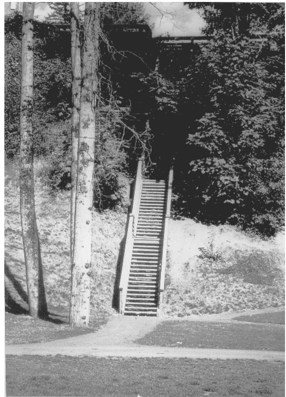
Figure 1.10. Access stairs at valley wall directly ascend the slope.
