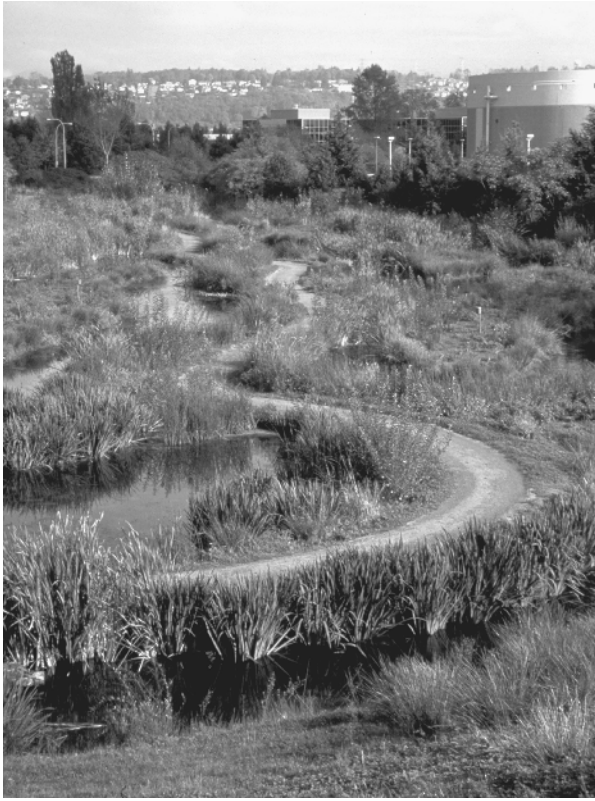
Figure 1.14. View across the wetlands shows the treatment plant in the background on the right. (Photo: Lorna Jordan)
