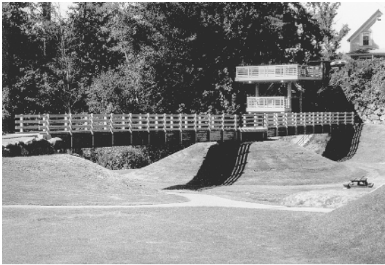
Figure 1.8. Bridge structure allows for greater water flow.
