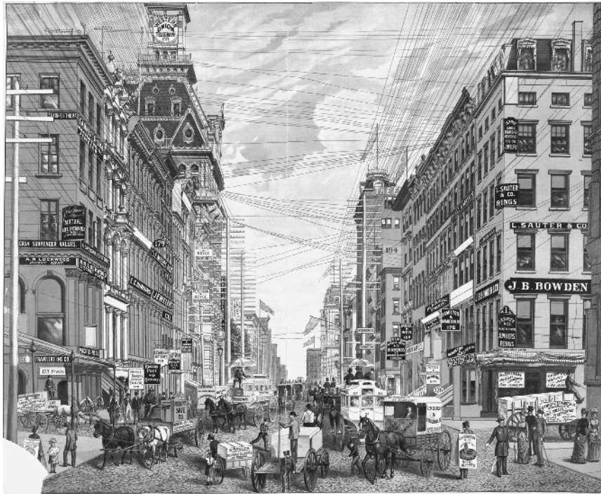
1.18 By 1890, community leaders had begun to argue for regulations to control the proliferation of telegraph, telephone, and electrical wires in Manhattan's streets. The city eventually required their burial, a precursor to broader controls that ultimately produced the country's first zoning ordinance. Courtesy Library of Congress, Prints and Photographs Division
