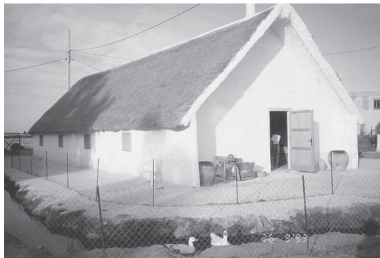
Figure 1.13 A wetland house in the Ebro River Delta region on the Mediterranean Sea, Spain. The walls are made from wetland mud, and the roof is thatched with reed grass and other wetland vegetation. (Photo by W. J. Mitsch)
