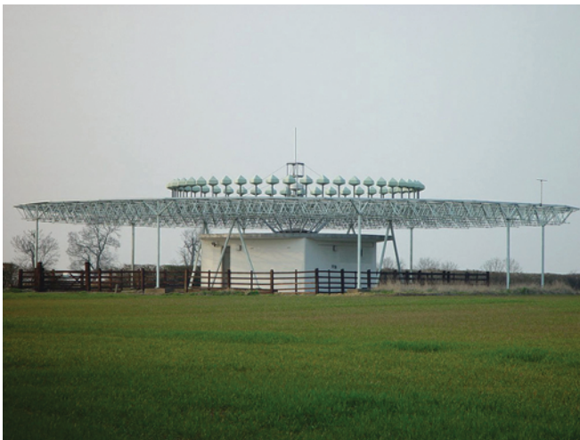
Figure 1.19 (a) The VOR transmits an omnidirectional signal with the same phase in all directions and a directional signal whose phase relative to the omnidirectional signal varies from 0 to 360° around the circle. The two signals are in phase along magnetic North. (b) The DTY VOR in the United Kingdom. Source: Photo reproduced with permission from Trevor Diamond ( http://www.trevord.com/navaids ).
