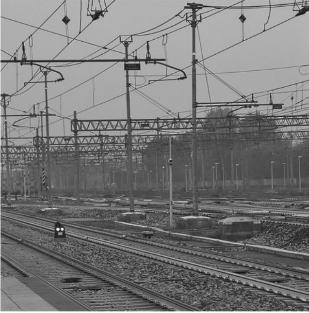
Figure 1.2 DC railway electrification system in Italy.
