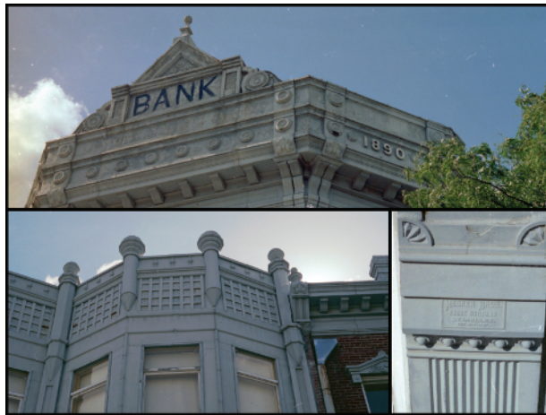
FIGURE 1.18 Mesker Brothers Kit Façade made of galvanized steel.
