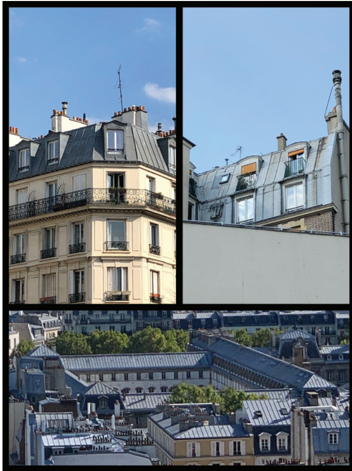
FIGURE 1.15 Zinc roofs in Paris.
