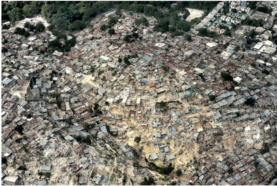
FIGURE 1.9B Aerial view of the destruction in downtown Port au Prince, Haiti as the result of the 2010 earthquake. Source: Courtesy of the USGS.
