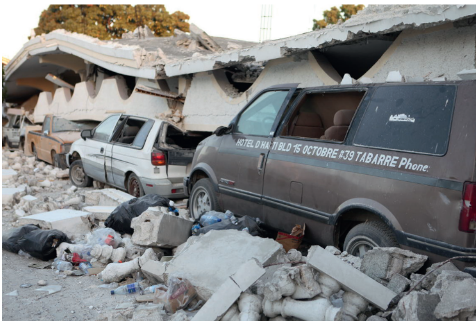
FIGURE 1.9A Collapsed buildings and crushed cars in Port-au-Prince, Haiti after the 2010 earthquake. Source: Courtesy of the USGS.
