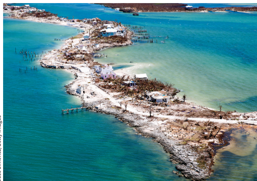
FIGURE 1.23B Great Abaco, Bahamas. Aerial view of the damage Hurricane Dorian caused. The hurricane hit Grand Abaco as a Category 5 storm. Its 20 foot storm surges leveled much of the northern Bahamas.
