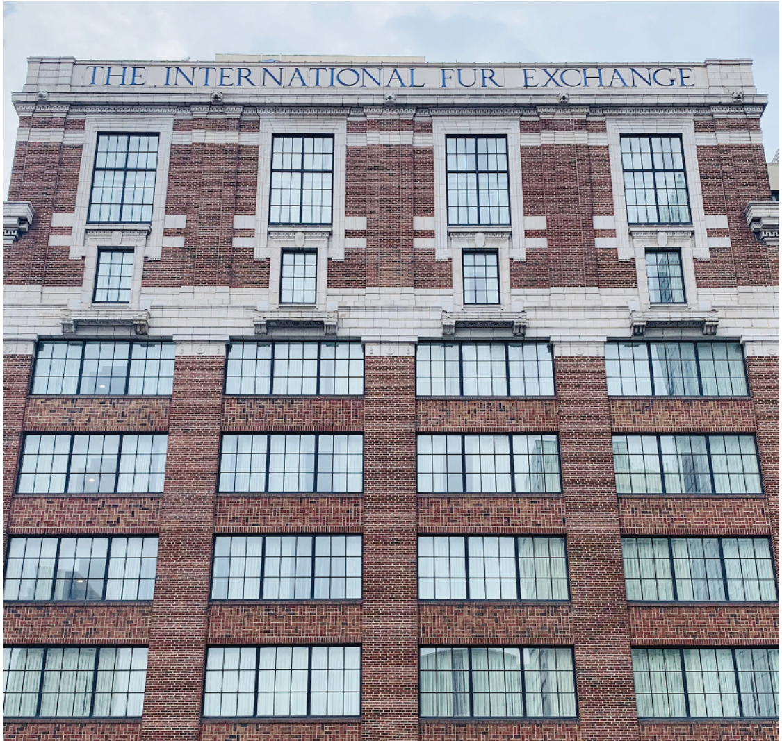
FIGURE 1.1 International Fur Exchange Building, St. Louis, Missouri, designed by Hellmuth & Hellmuth. Source: Photo courtesy of HOK.
