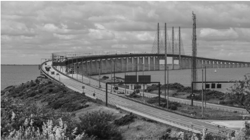
Øresund Bridge. Source: reduper.com
