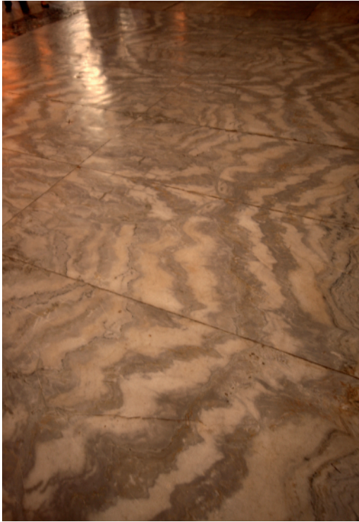
Detail of Proconnesian marble floor, Hagia Sophia, Constantinople (Istanbul), from AD 360 Paul the Silentiary's 6th-century description of the ambo – 'And as an island rises amidst the waves of the sea' – suggests the metaphor of the frozen sea evoked so clearly by the slabs of Proconnesian marble.
