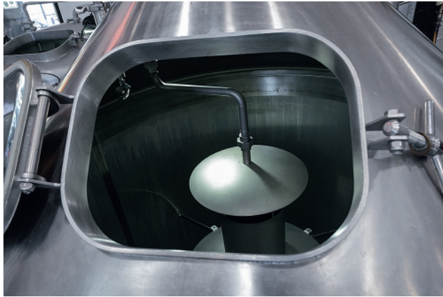
Figure 1.6 Brew kettle at Bonesaw Brewing showing internal calandria. Source: Photo by Naomi Hampson.
