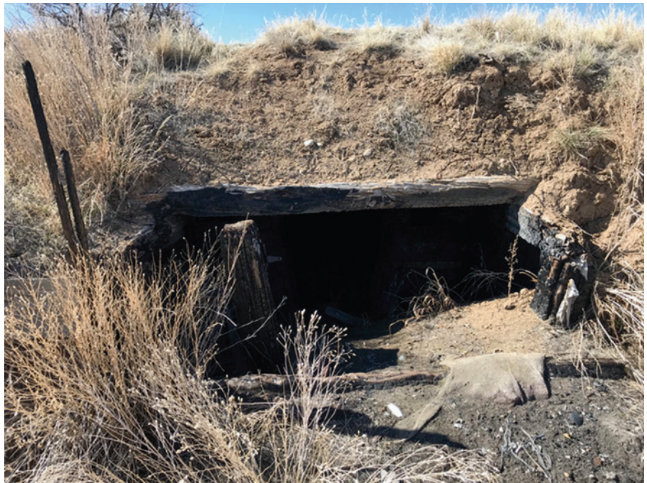
Figure 1.2 A century old hand-dug cellar near Arapahoe, WY, USA. This is an early example of a much-decayed storage cellar. Colonies of bees were hand carted into the cellar for winter. Ventilation pipes (no longer visible) brought in fresh air and a primitive chimney exhausted air for "circulation." Cellar dug by Lawrence George Krause. Source: Photo by John Miller.
