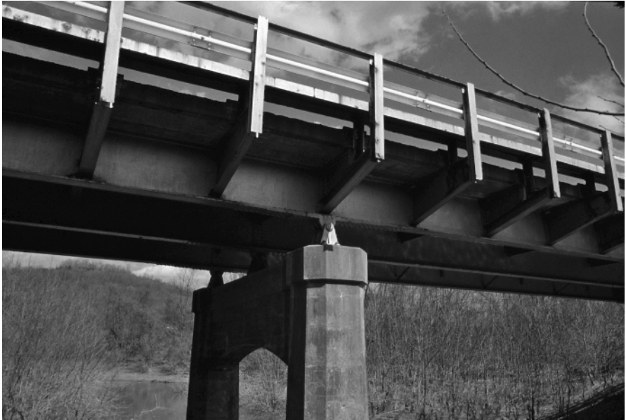
Figure 1.1 USR 52, Isaacs Creek Bridge, Adams County, Ohio, 1931. This was one of first steel beam bridges in Ohio where riveted field splices at piers were used to achieve superstructure continuity.
