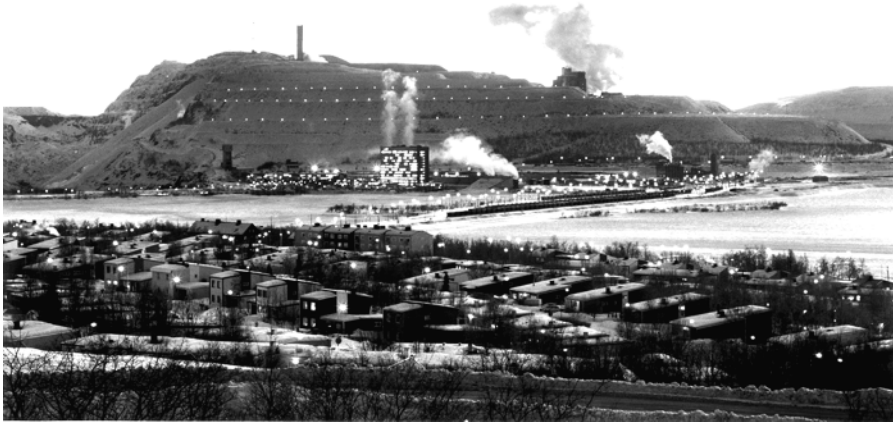
Figure 1.8 Kirunavaara iron ore mountain, northern Sweden. The steeply dipping magnetite orebody was originally mined in an open pit on the left side of the hill. Today, extraction is underground. Courtesy LKAB 2010.
