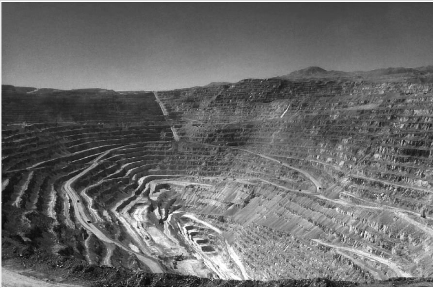
Figure 1.31 (Plate 1.31) Chuquibambilla open pit in Chile, one of the world's largest porphyry copper mines. Courtesy Bernd Lehmann, Clausthal. The pit measures 2 × 3 km and approaches a depth of 900 m. Total pre-mining resources were nearly 3000 Mt at 1% Cu and by-product Mo. Annual production is ~1.2 Mt copper and 20,000 t molybdenum plus rhenium.
