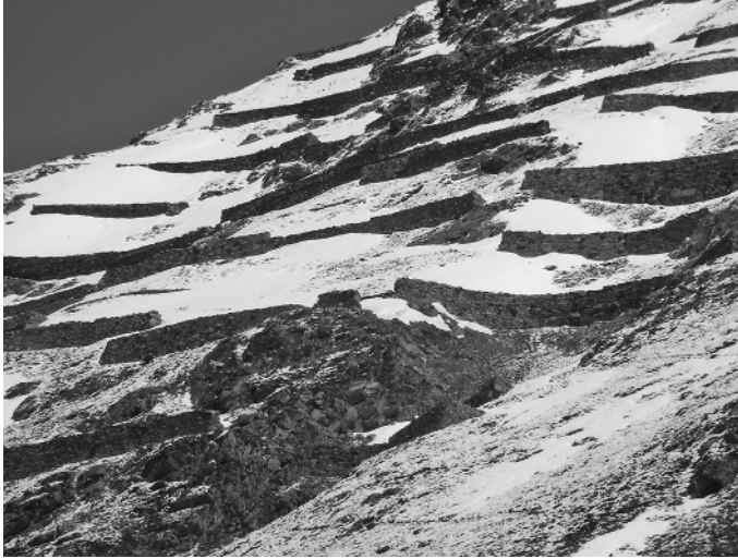
Fig. 1.10 Historical avalanche defense structures: rock fill terraces at the Schafberg mountain in Pontresina (Switzerland), constructed around 1900 (© Margreth)
