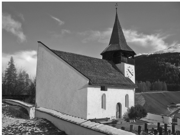
Fig. 1.9 Historical avalanche defense structures: Endangered by the avalanche Frauentobellawine, the church Frauenkirche was protected by an avalanche splitting wedge, constructed most probably in the 16th century (© Margreth)
