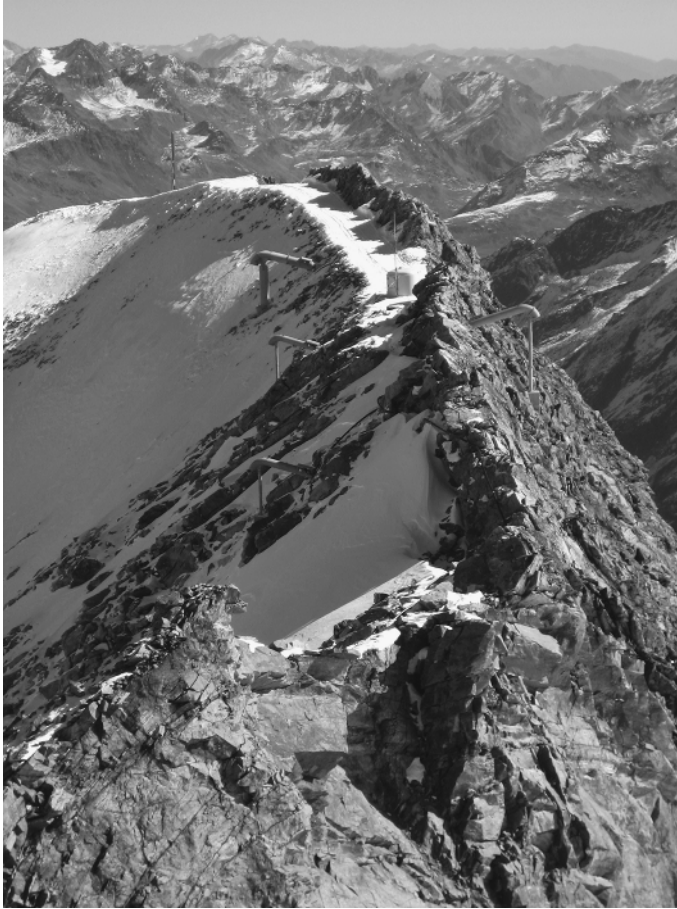
Fig. 1.6 Artificial avalanche release facilities with the system Gaz.Ex (© Interfab Snowbusiness GmbH)
