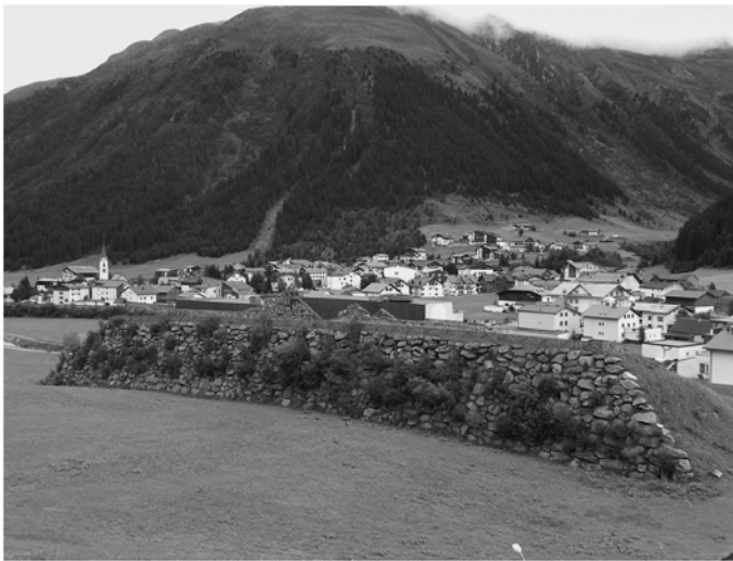
Fig. 1.5 Examples of structural avalanche defense structures: (a) snow nets in a starting zone (© Sauermoser); (b) avalanche retarding dam in the municipality of Galtür (Tyrol) (© Rudolf-Miklau)
